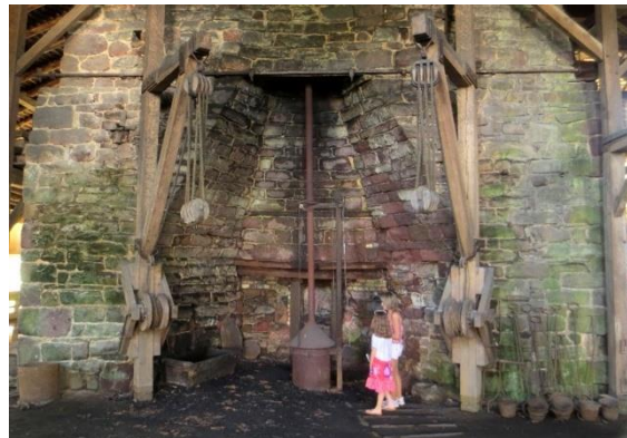
Restored Furnace Stack in the Casting House
